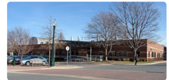
US Pharmacopiea renewal - 25,000 sf at 12725 Twinbrook Avenue.
